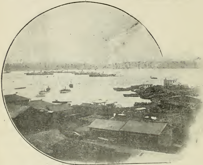
Port of Mororan and the Co.'s head office.
